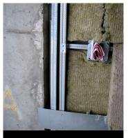
Make sure that the hard to get to areas are filled prior to the final install of the studs or metal backing.
