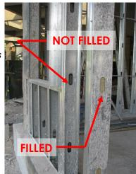
Framing columns were installed with insulation, however, the double stud at the window was not. Also, the holes need to be covered for exterior exposure.
